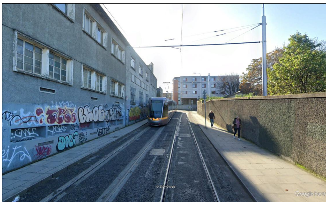
Figure 6. LUAS Service on Steeven's Lane
