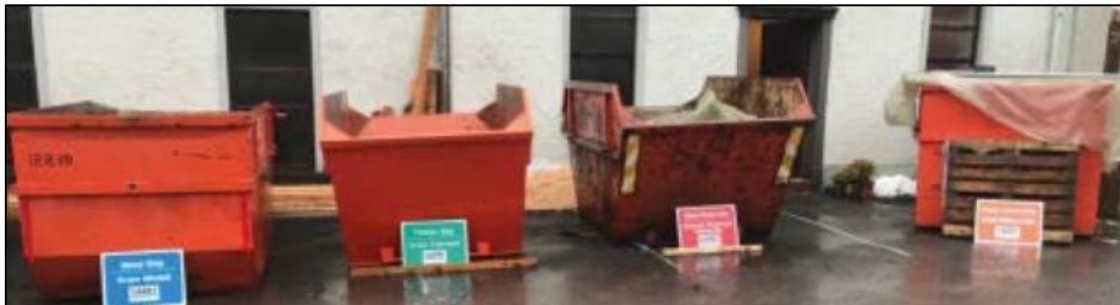
Figure 8-1: Good Practice Waste Segregation (Source: EPA RWMP Guidelines)
